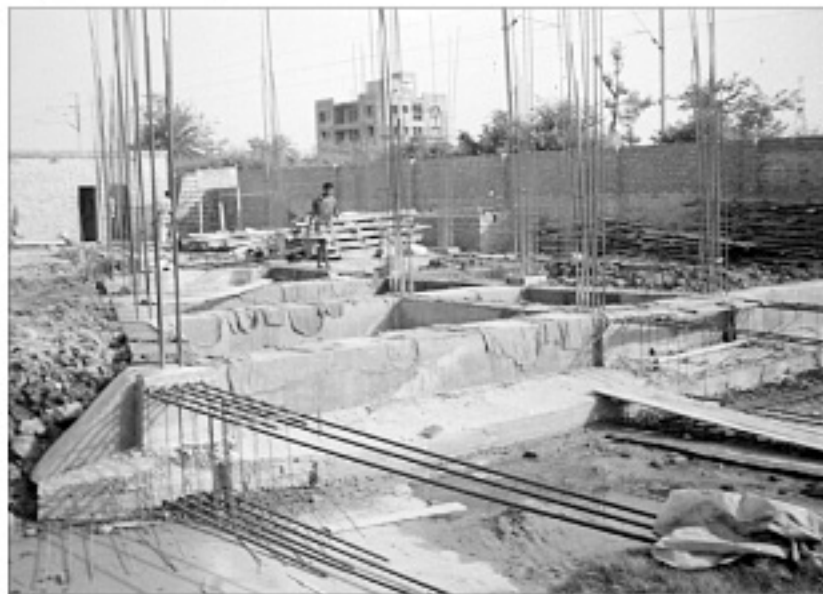
Foundation for new Paripurnata building
